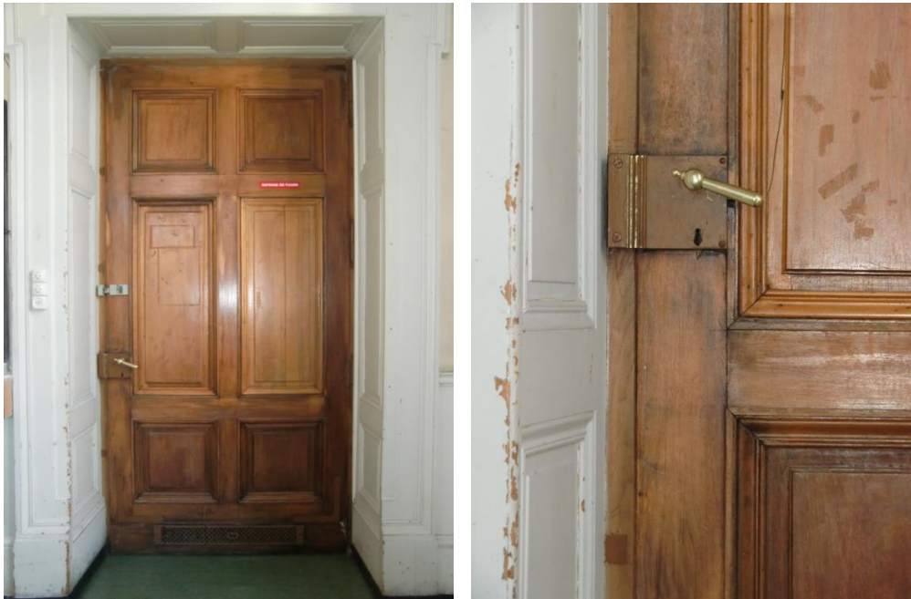
Figure 3. Historic doors and detail of fixtures used at the Bastions Building, University of Geneva
